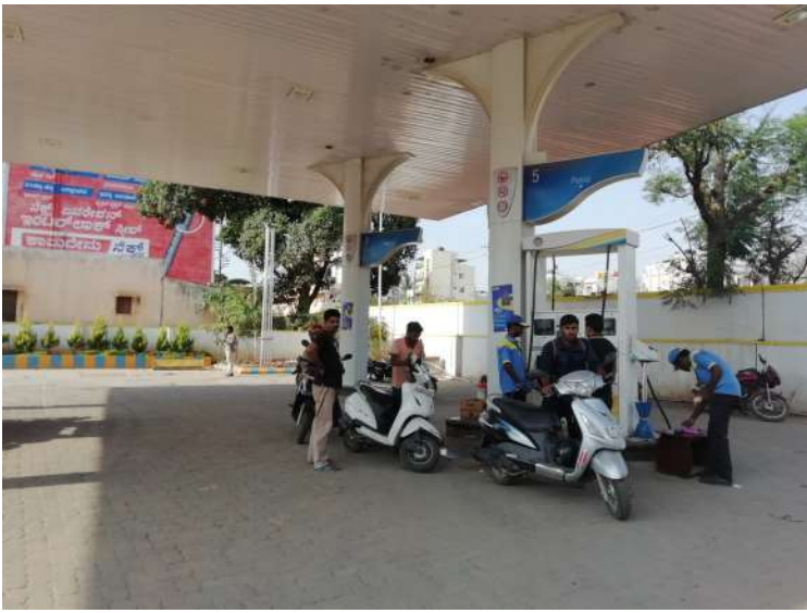
Patel Service Station, Bangalore
